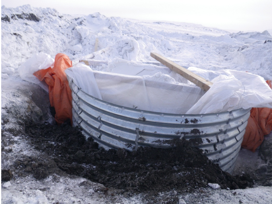
Photo 5: Sump – Overburden material in the annulus of sump 2.
