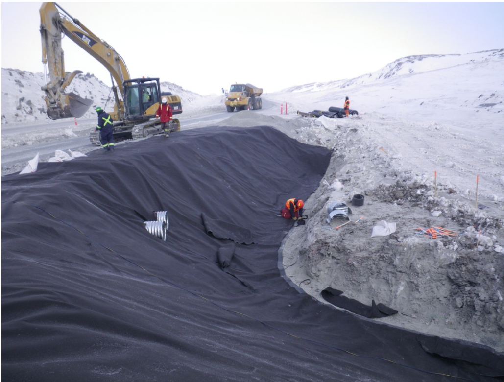
Photo 4: Diversion Berm – View of geotextile placed in the corner near the start of the diversion berm alignment.
