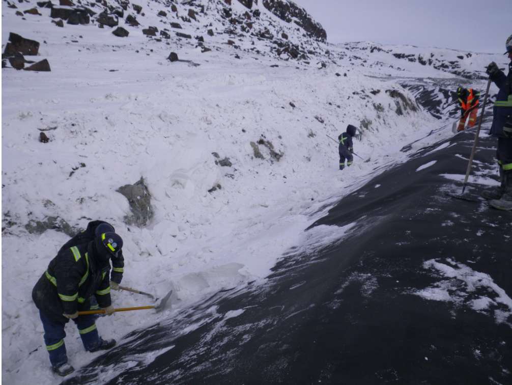
Photo 7: Diversion Berm – Labourers cleaning snow from the geotextile and liner.
